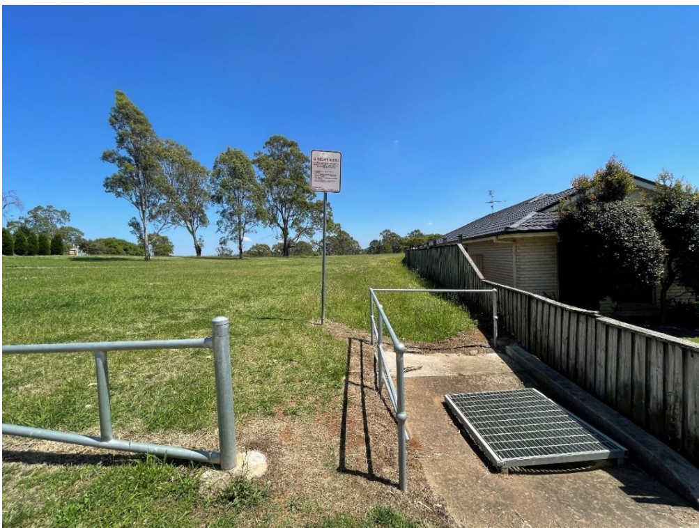
Photo 2: View (southeast–northwest) from Glendower Street to the west boundary of Lot 19. Note a stormwater drain located at the eastern corner of Lot 19 behind residential properties. Also, note scattered medium-size trees within Lot 19.
